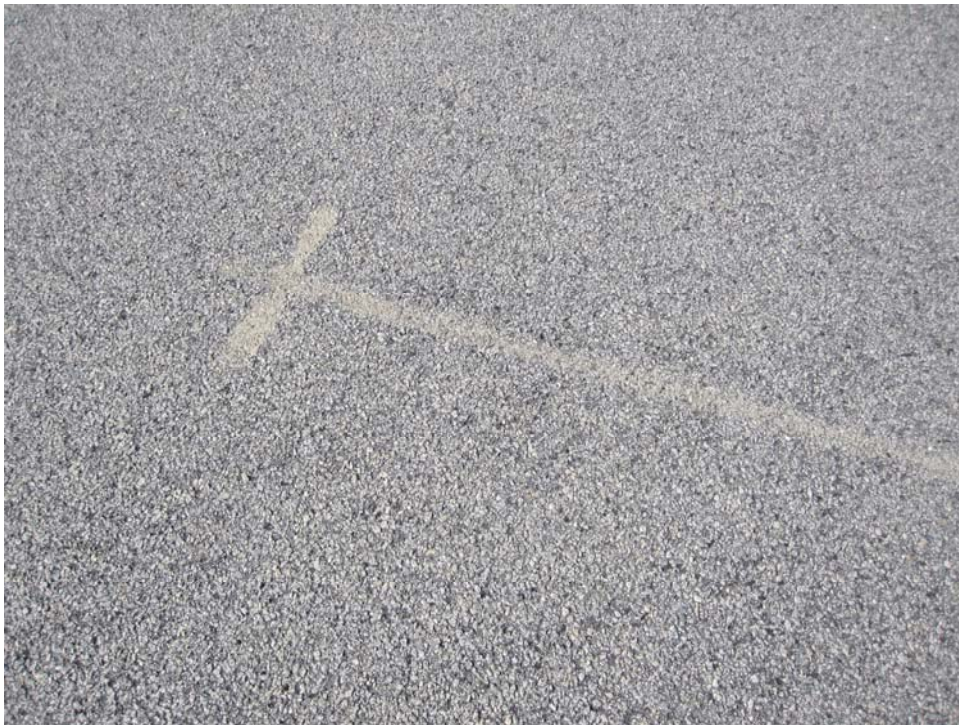
THANGAG-10. Unsatisfactory Paint.
