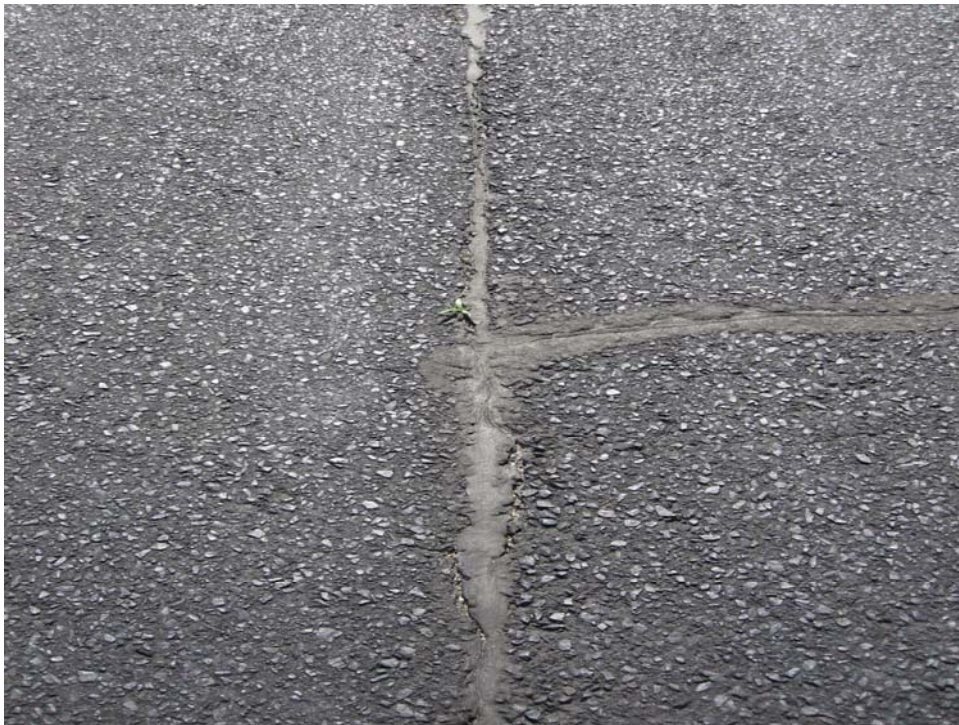
ATERMAG-30. Longitudinal and Transverse Cracking (Sample Unit #33).
