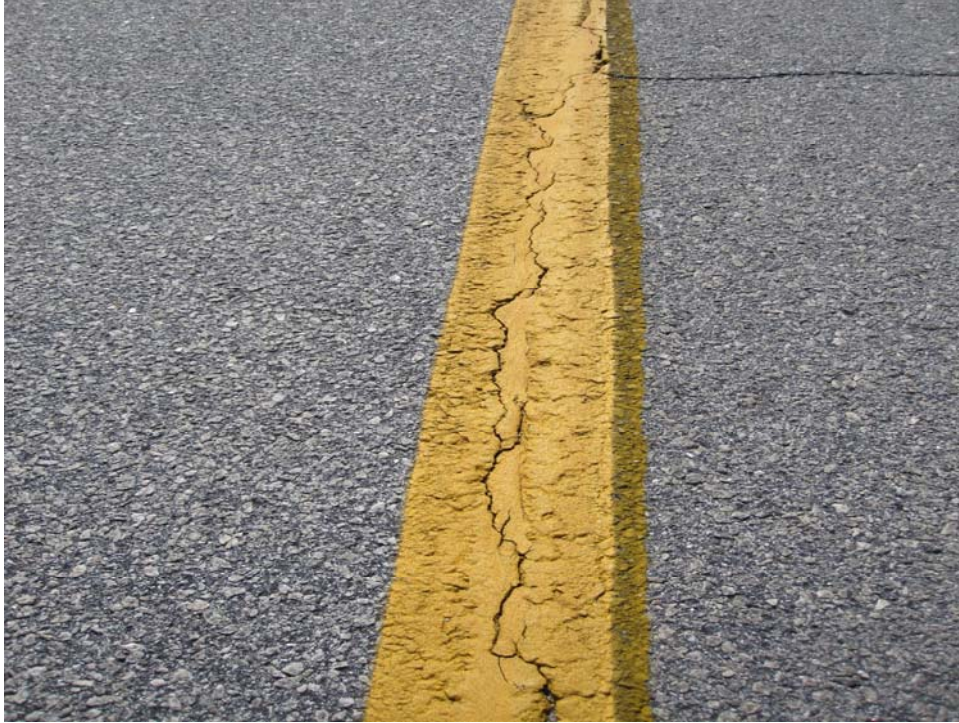
TDAG-10. Longitudinal and Transverse Cracking (Sample Unit #22).
