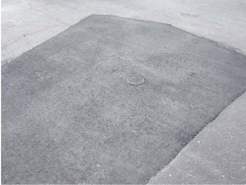
ATERMAG-10. Patching (Sample Unit #01).
