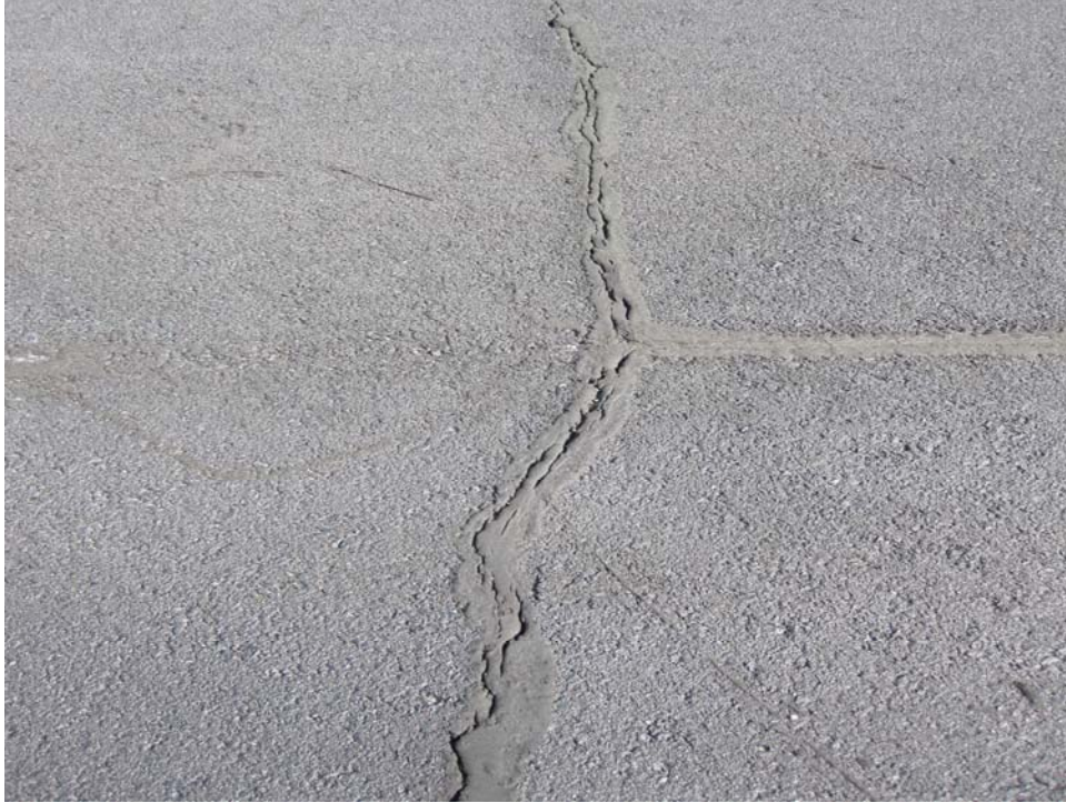
R1129AG-10. Longitudinal and Transverse Cracking (Sample Unit #09).
