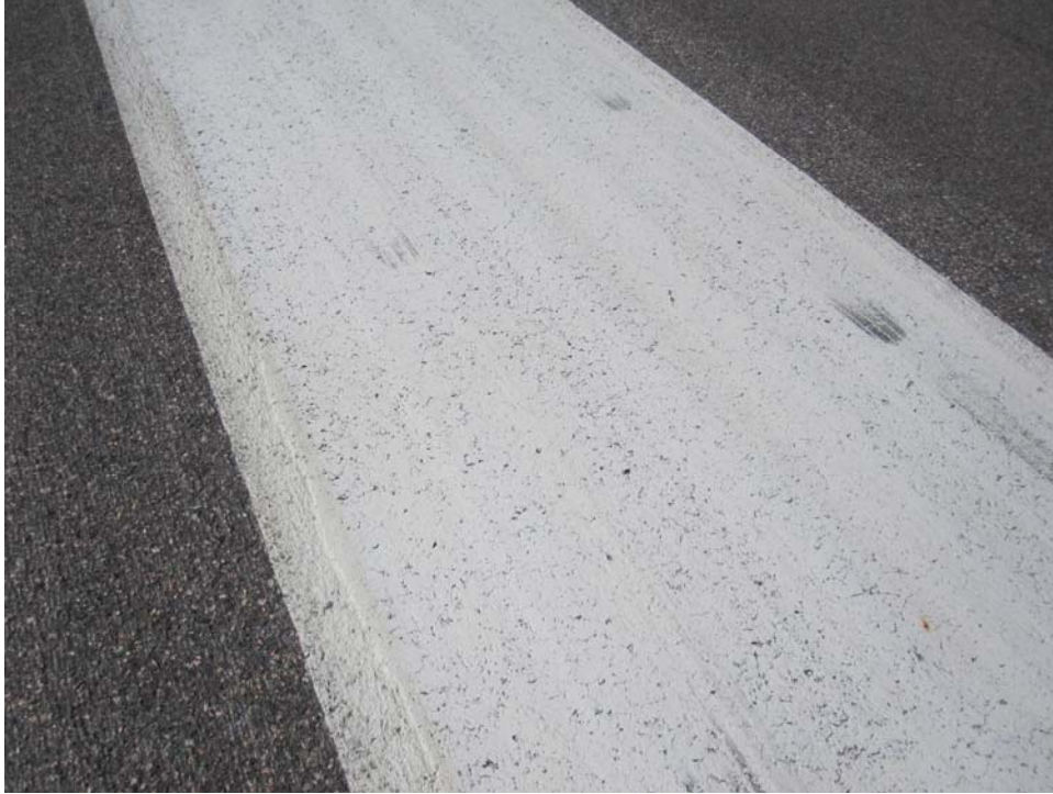
R0523AG-20. Satisfactory Paint.
