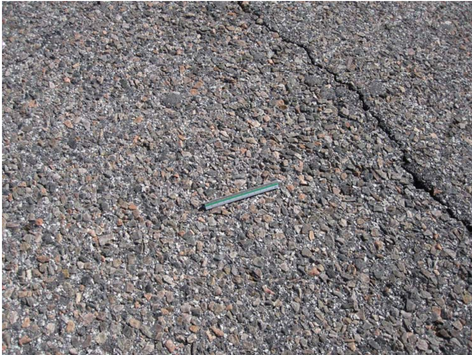
R0523AG-10. Weathering (Sample Unit # 06).
