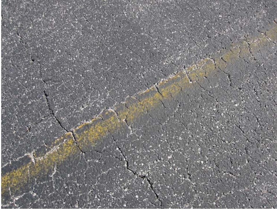
ATERMAG-40. Unsatisfactory Paint.
