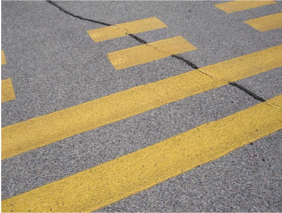
ATOWERAG-20. Satisfactory Paint.
