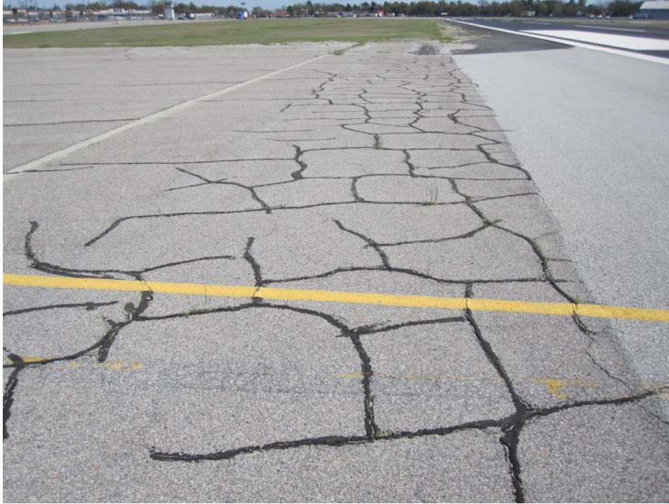
ATOWERAG-20. Block Cracking (Sample Unit #03).
