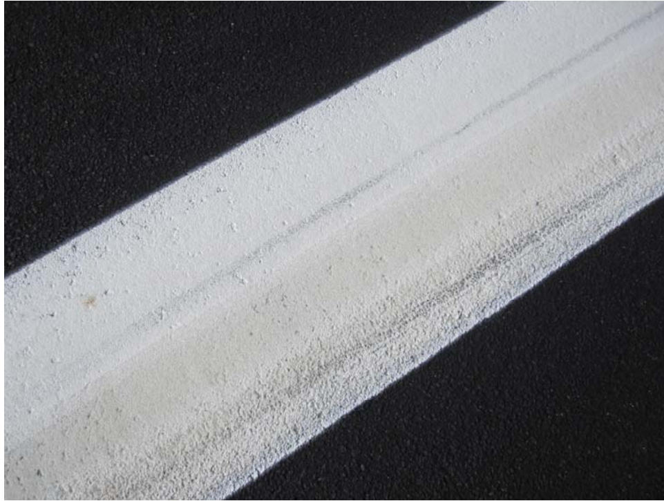
R1129AG-10. Satisfactory Paint.
