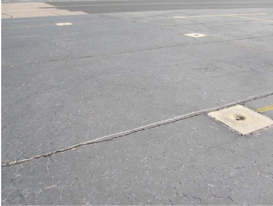
ATERMAG-30. Raveling (Sample Unit #39).
