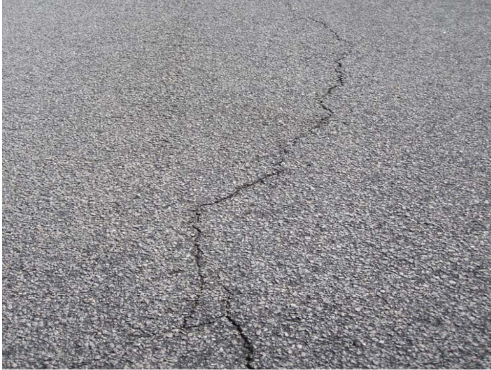
THANGAG-10. Longitudinal and Transverse Cracking (Sample Unit #08).
