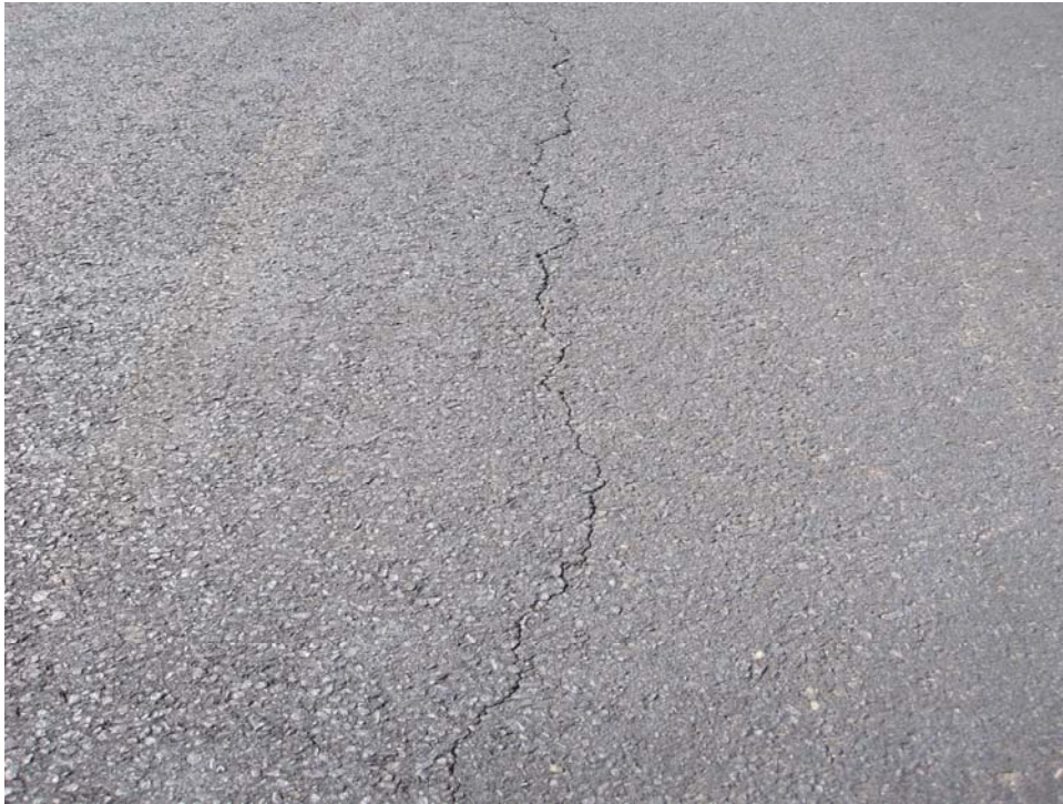
R0523AG-20. Longitudinal and Transverse Cracking (Sample Unit #04).
