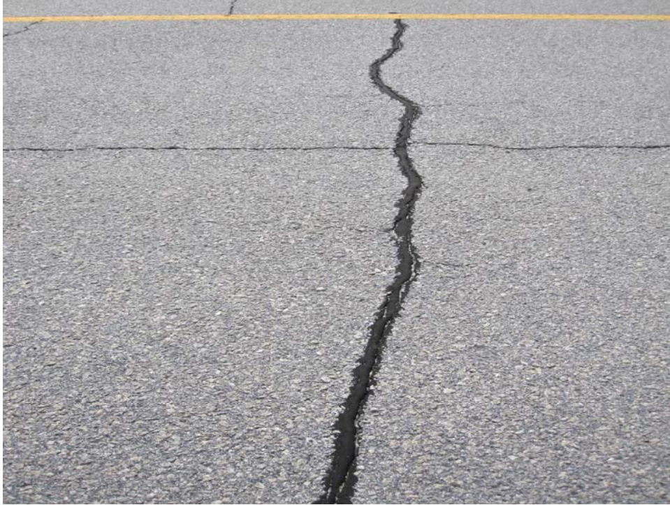
TAAG-10. Longitudinal and Transverse Cracking (Sample Unit #16).
