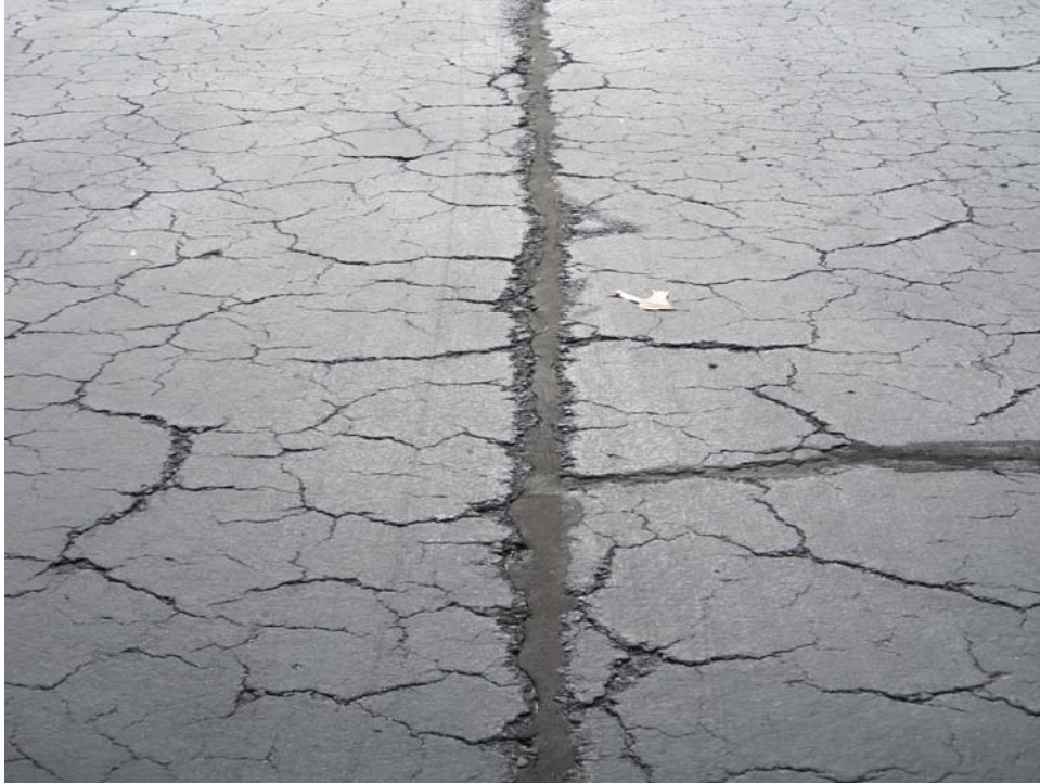
ATERMAG-30. Longitudinal and Transverse Cracking (Sample Unit #19).
