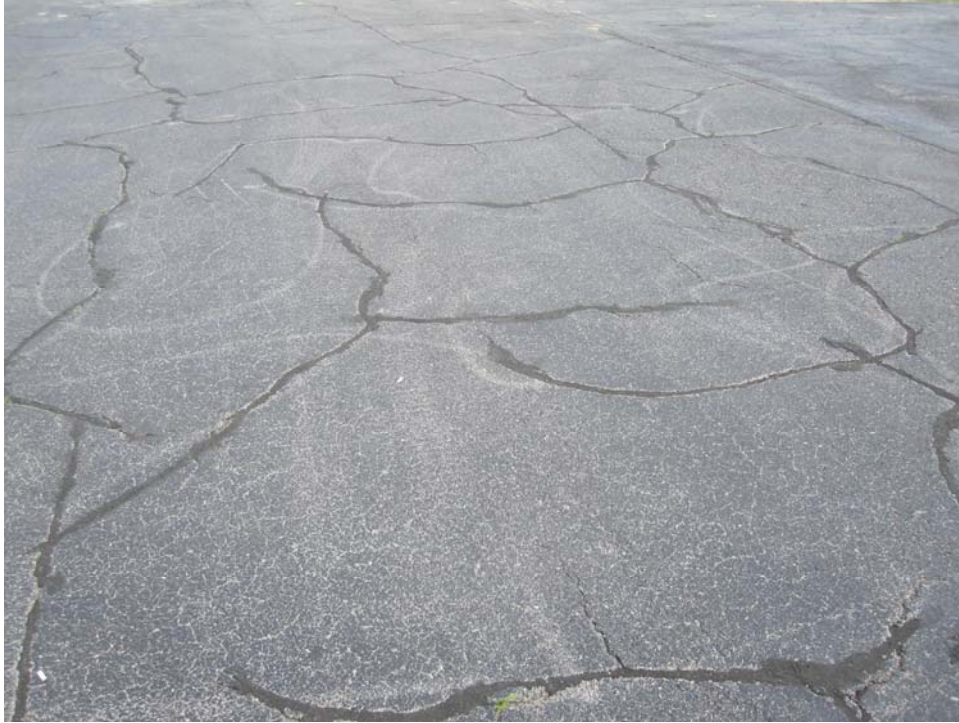
ATERMAG-70. Block Cracking (Sample Unit #01).
