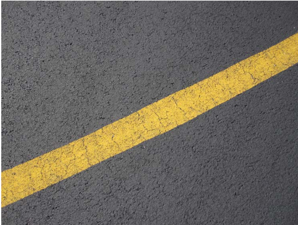
ATERMAG-10. Satisfactory Paint.
