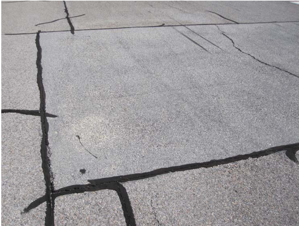
R0523AG-10. Patching (Sample Unit #15).
