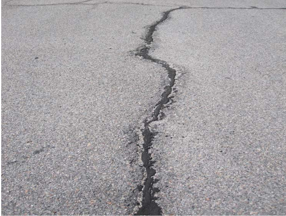
ATOWERAG-10. Longitudinal and Transverse Cracking (Sample Unit #01).
