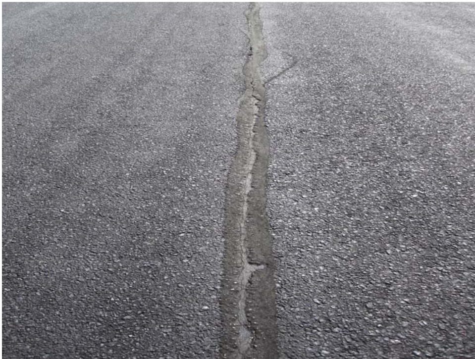
R1129AG-10. Longitudinal and Transverse Cracking (Sample Unit #22).
