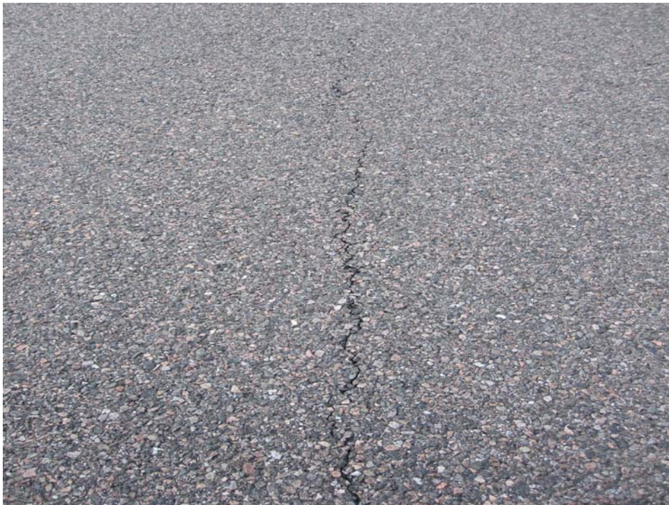
TEAG-10. Longitudinal and Transverse Cracking (Sample Unit #01).
