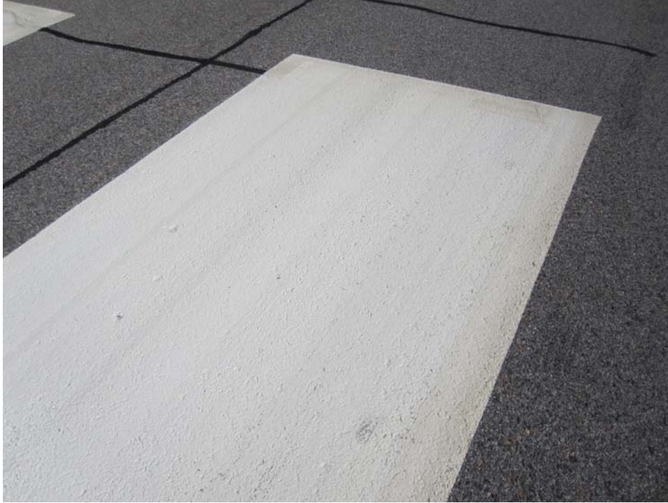
R0523AG-10. Satisfactory Paint.
