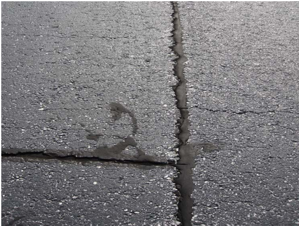
ATERMAG-40. Longitudinal and Transverse Cracking (Sample Unit #11).
