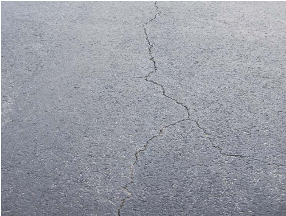
ATERMAG-20. Longitudinal and Transverse Cracking (Sample Unit #05).
