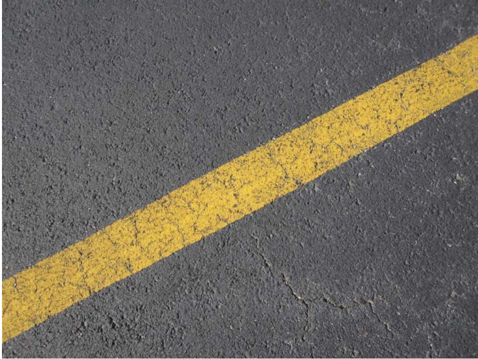
ATERMAG-20. Satisfactory Paint.
