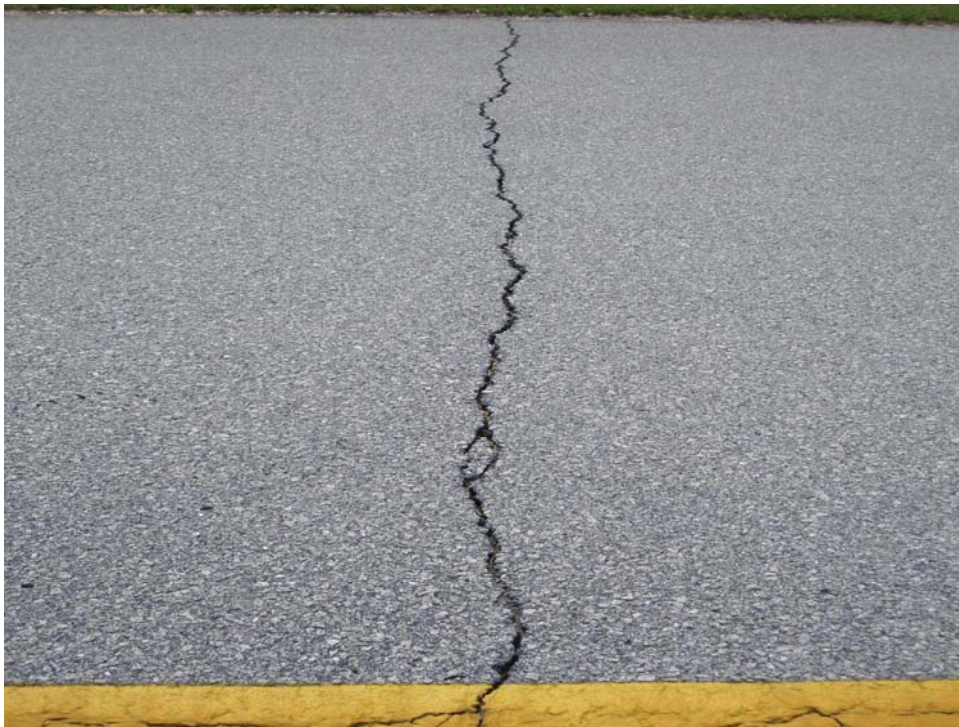
TAAG-10. Longitudinal and Transverse Cracking (Sample Unit #05).
