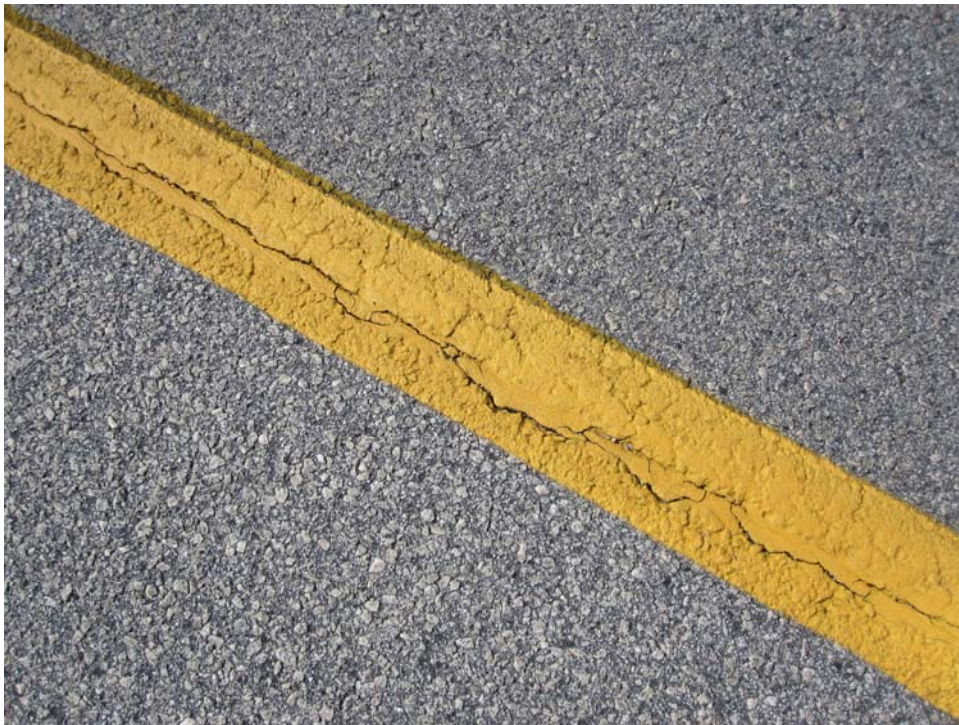
TDAG-10. Satisfactory Paint.
