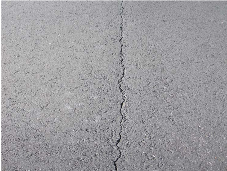
ATERMAG-10. Longitudinal and Transverse Cracking (Sample Unit #13).
