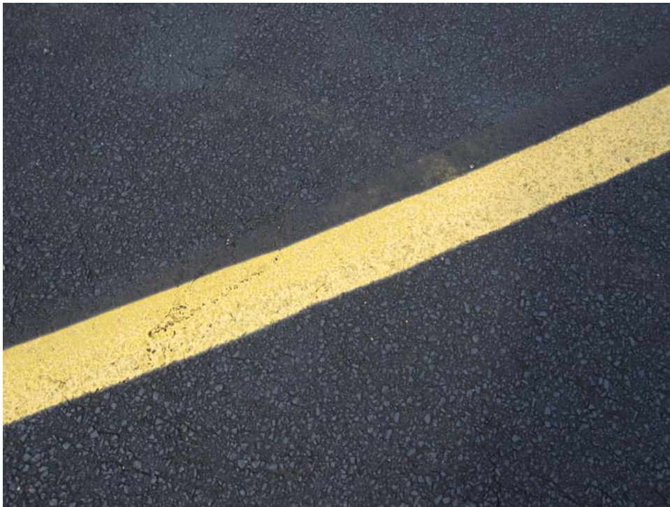
ATERMAG-30. Satisfactory Paint.
