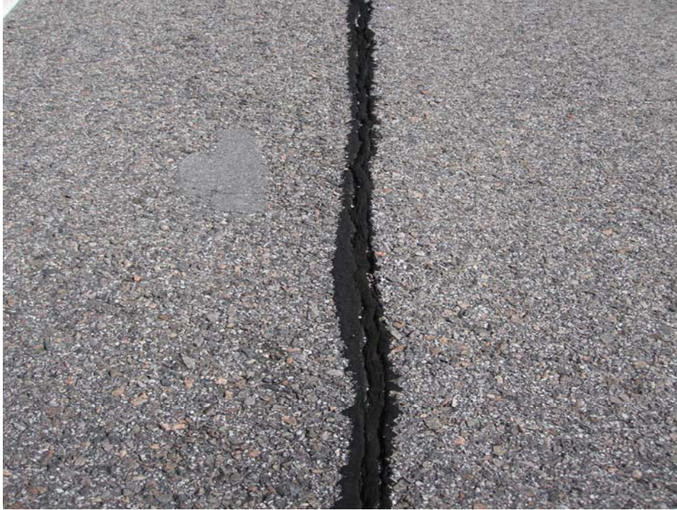
R0523AG-10. Longitudinal and Transverse Cracking (Sample Unit #06).
