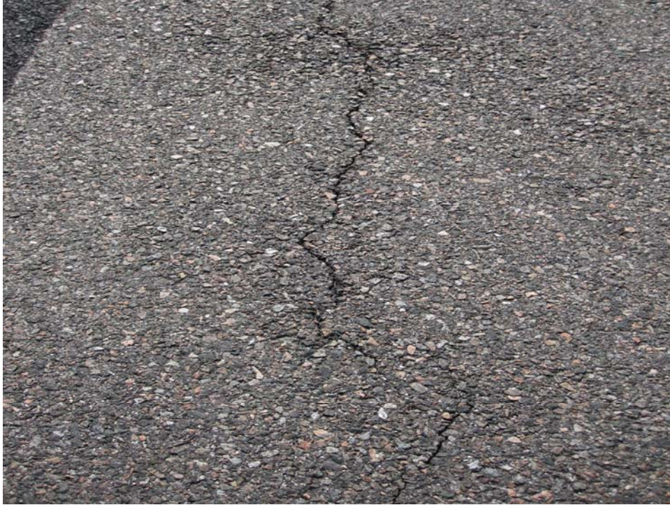
ATERMAG-60. Longitudinal and Transverse Cracking (Sample Unit #03).
