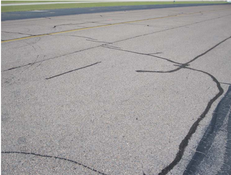
ATERMAG-30. Weathering (Sample Unit #49).
