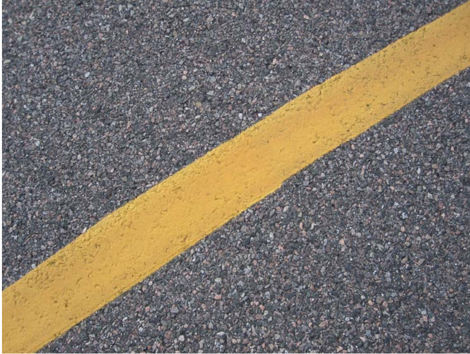
TEAG-10. Satisfactory Paint.
