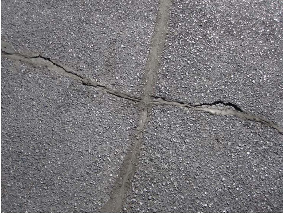
ATERMAG-50. Longitudinal and Transverse Cracking (Sample Unit #10).
