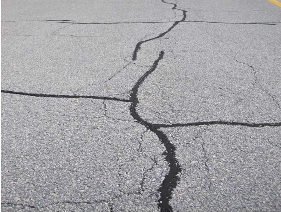
TAAG-10. Alligator Cracking (Sample Unit #05).
