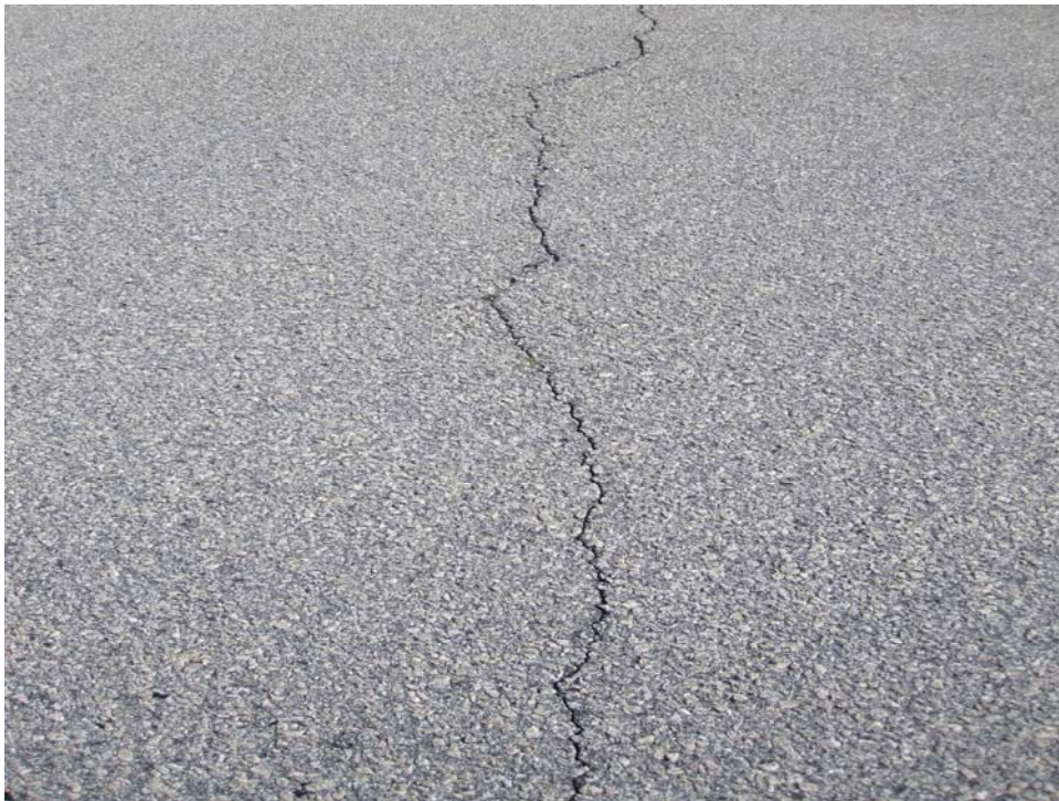
TDAG-10. Longitudinal and Transverse Cracking (Sample Unit #18).
