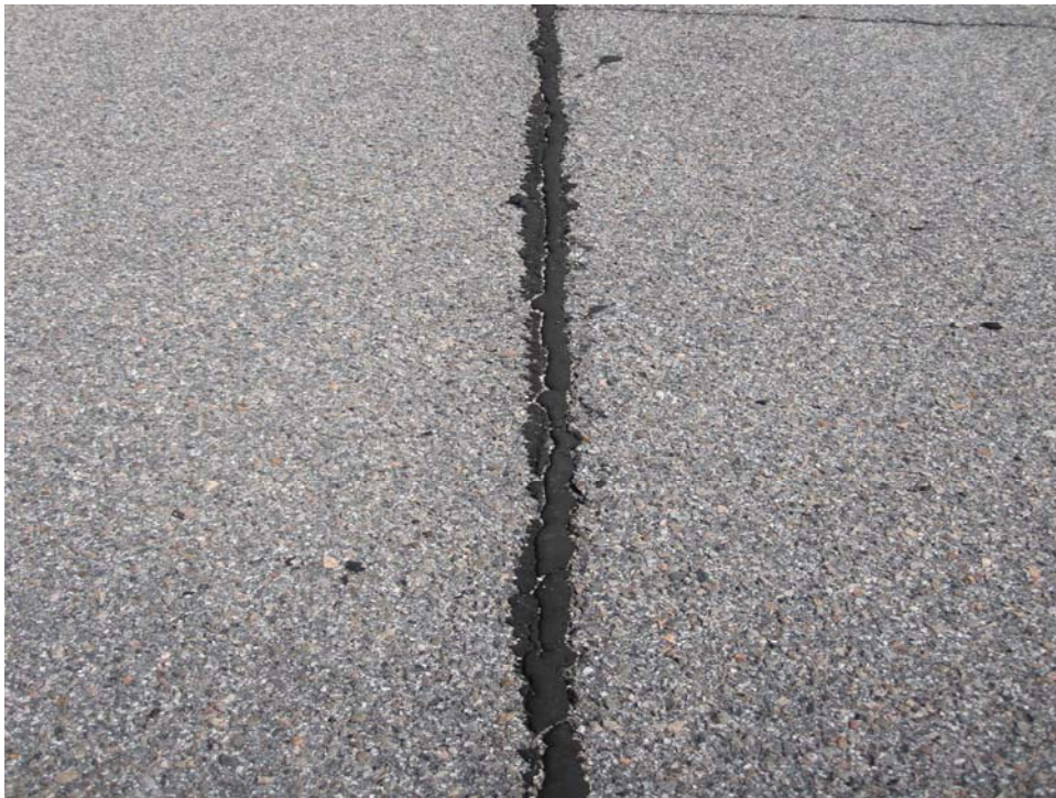
ATOWERAG-20. Longitudinal and Transverse Cracking (Sample Unit #23).
